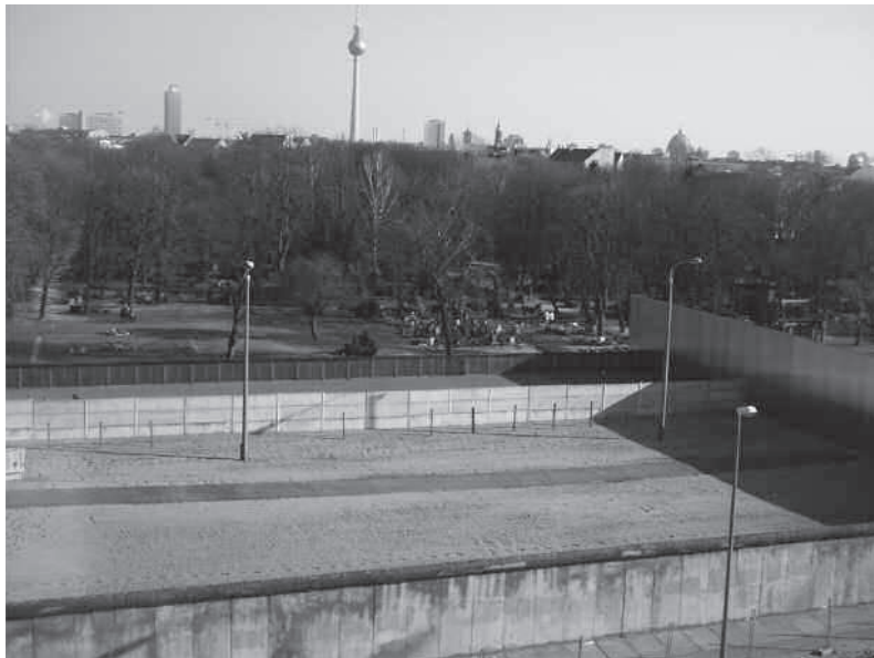
Fig. 4.6. Museumification of the Berlin Wall at the Bernauerstrasse.
